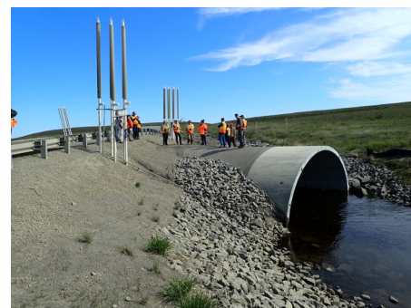
"The Gunghi Creek crossing on the Inuvik-Tuktoyaktuk Highway". This photo is associated with the 2025 Inuvialuit Permafrost Workshop story.
