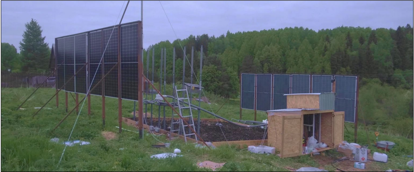
Figure 6. Construction of the winter road site.
