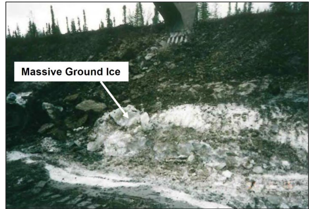
Figure 4. Massive ground ice exposed during excavation of borrow material in 1995.
