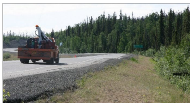
Figure 4. Localized thaw subsidence zones along the Dalton Highway, Alaska, USA, due to the degradation of ice wedges.
