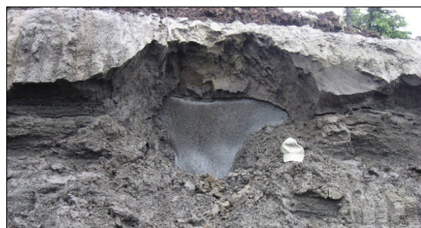
Figure 3. Ice wedge exposed in a road cut along the Dalton Highway, Alaska, USA. The baseball cap on the right provides the scale. All copyrights reserved to AKDOT.
