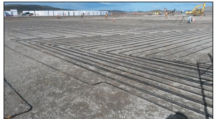
Figure 3. Evaporator installation at the ATB. Rigid insulation is stockpiled in the background.
