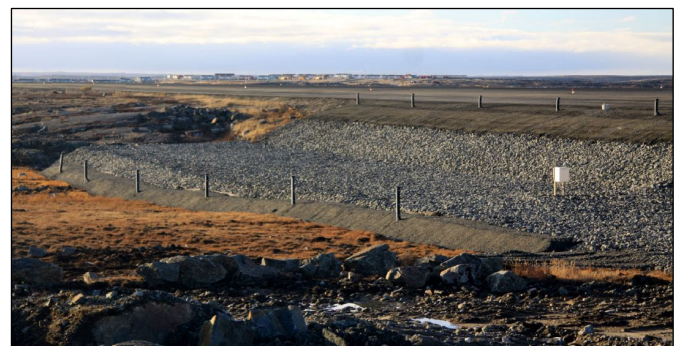
Figure 8. Application of ACE at Puvirnituk airstrip, Nunavik, Québec.
