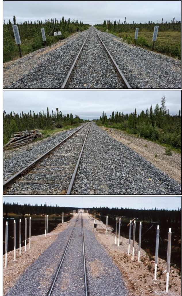
Figure 3. Mitigation techniques designed and tested along the Herchmer Subdivision between Gillam and Weir River from 1976 to 1991. Top images: 800 Cryo-Anchor heat pipes and 6H:1V gentle slope with wood chips insulation. Bottom image: Thermo-probes.
